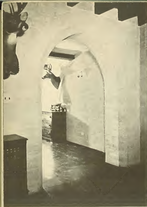
Random concrete ashlar, painted in light colors, forms the walls of this basement recreation room in a Detroit home.
